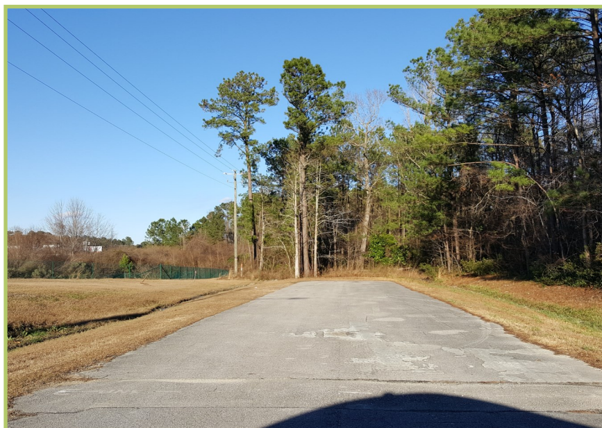
Facing east at start of STIP Project.
